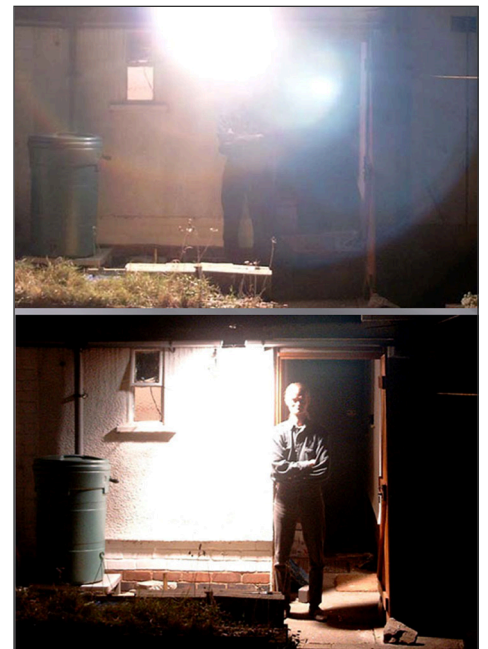
Fully shielded lighting is safer, more efficient, and costs no more than non-shielded lighting
